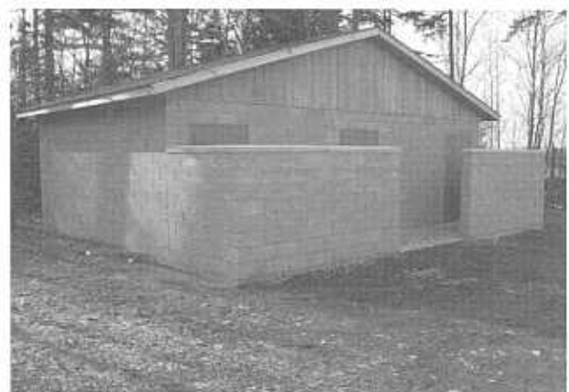
The new Recreation restroom building (sans paint) was built near the soccer field, track, picnic shelter, and skate park. The building cost the General Fund approx. $58,000, including the sewer line extension.
